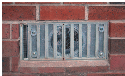
Installed behind existing vent
